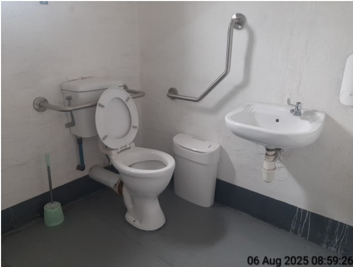
female toilet and wash basin
